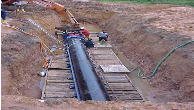
Typical Layout of an Entrance Pit for Thrustboring Operation @ Aluu, Rivers State.
