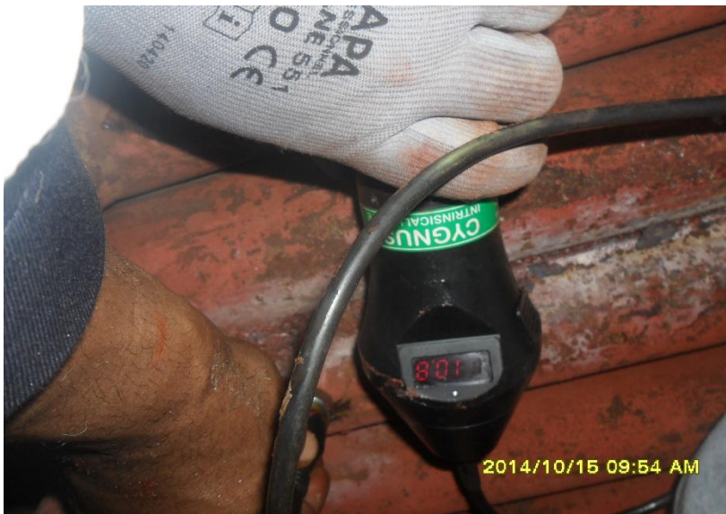
SPORT CHECK ON SELECTED PIPES
