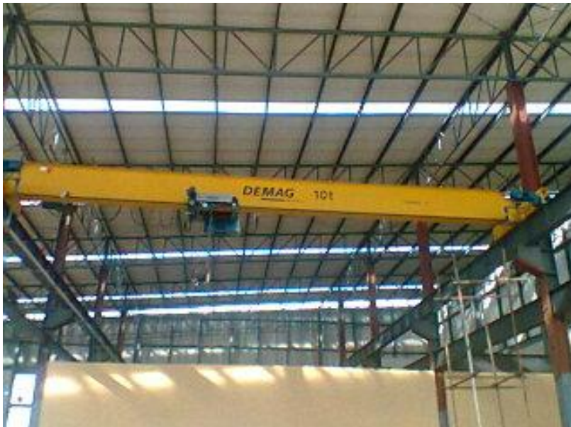
INSTALLATION OF 10TONS OVER HEAD CRANE AT PETROCHEMICAL
